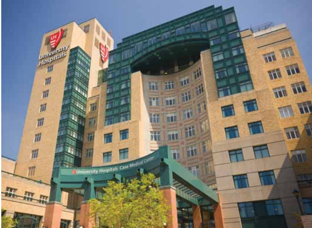
The Alfred and Norma Lerner Tower at University Hospitals Case Medical Center
